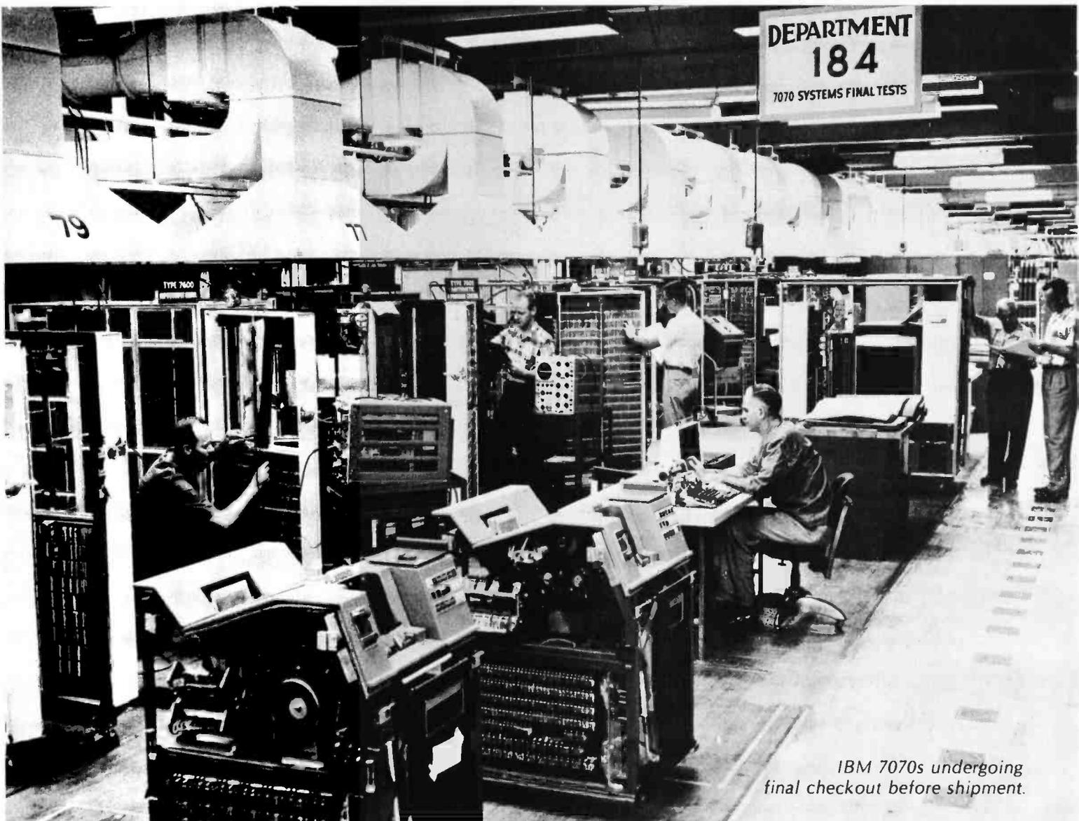
*IBM 7070s undergoing final checkout before shipment.*
